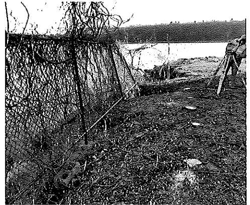
Site survey conducted prior to stabilization
