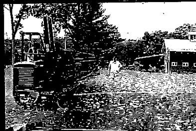
Delivery of original rafters
