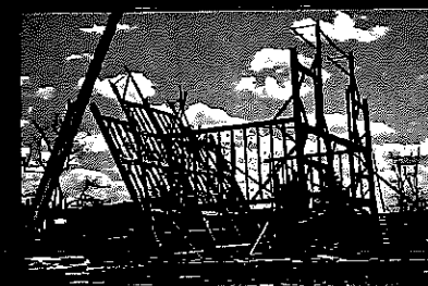
Bent 4 rising into place
