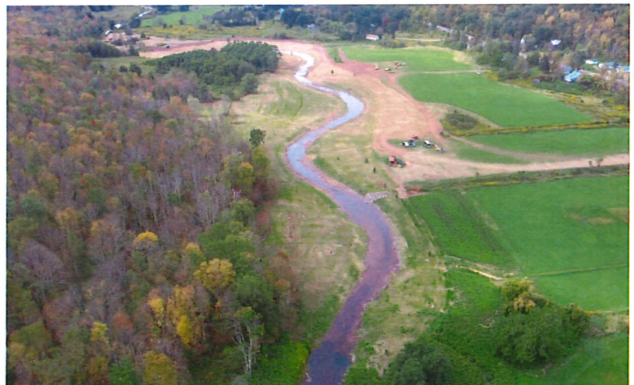
The Batavia Kill after completion of the project in fall 2017.
