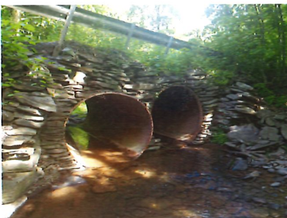
Left: The original metal double culvert.
