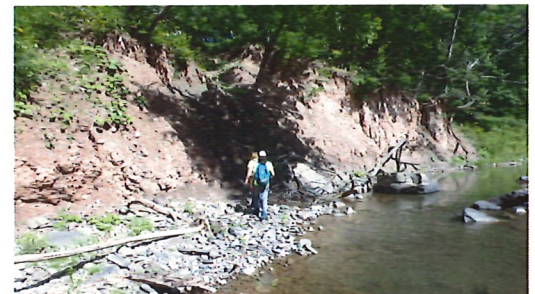
The lack of vegetation on the bank and leaning trees at the top are both signs of active erosion.
