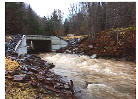
Right: Completed culvert
