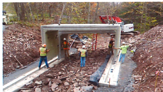
Center: Installation of the new concrete box culvert.
