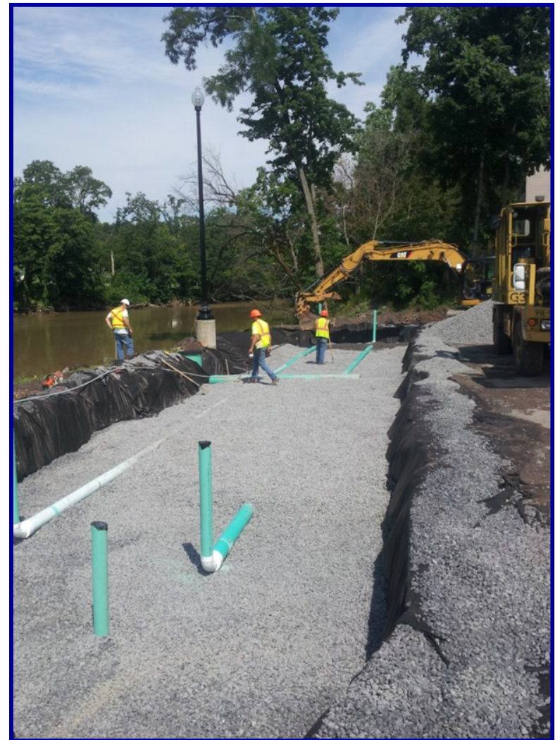
During the Construction of Phase 2, Slope Stabilization and Infiltration Bed Project
