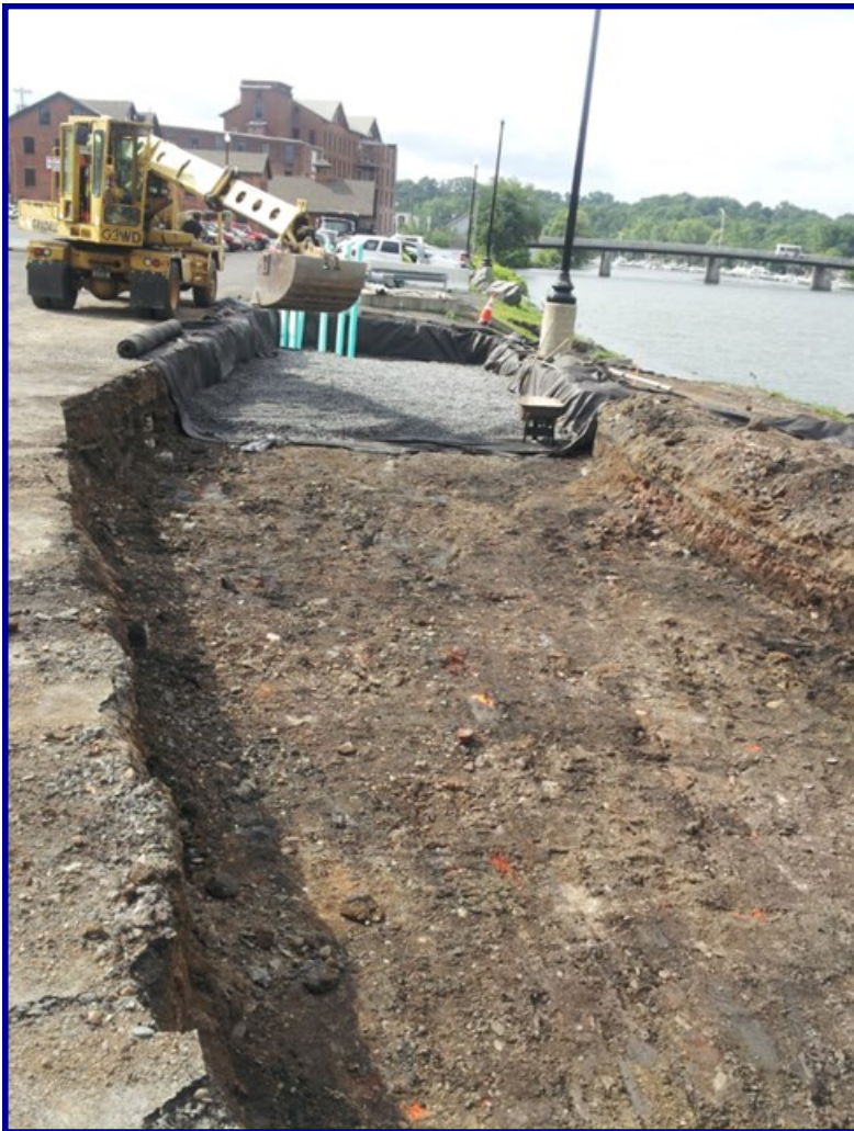
During the Construction of Phase 2, Slope Stabilization and Infiltration Bed Project
